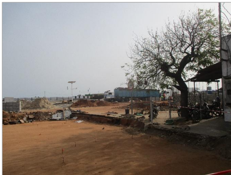
Photo 4: Demolition and reconstruction operations at the Sanvée-Condji/Hilla-Condji OSBP at the Togo/Benin border
